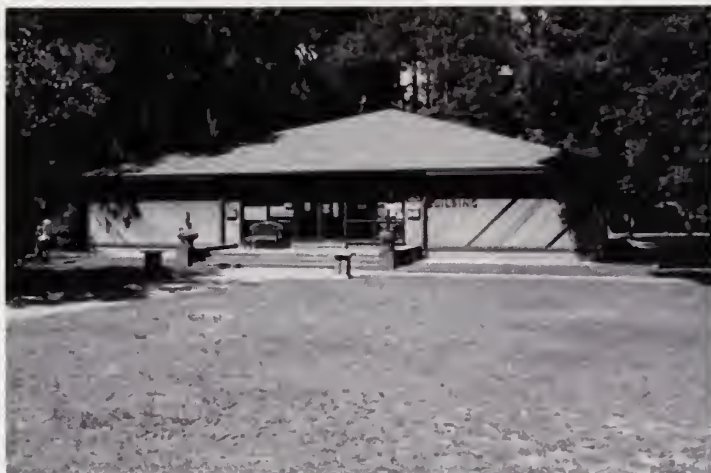
FIGURE 37. Lost Colony Activities Building. Source: JMA, Inc., 2009.
