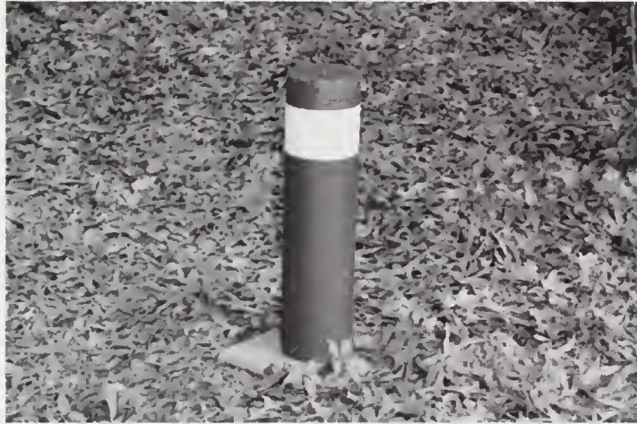
FIGURE 77. Small metal bollard light located throughout the visitor center area of the park. Source: JMA, Inc., 2009.
