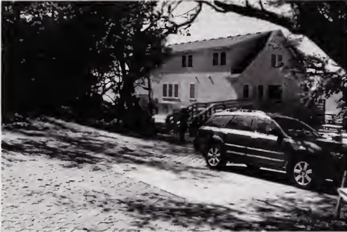
FIGURE 43. The recently-constructed Costume Shop. Source: JMA, Inc., 2009.
