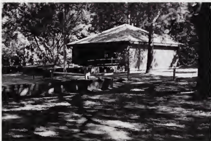
FIGURE 38. Restroom building. Source: JMA, Inc., 2009.
