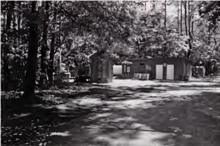
FIGURE 44. Buildings and utilities at the Water Plant. Source: JMA, Inc., 2009.
