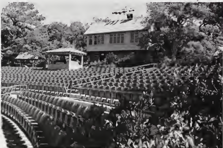
FIGURE 42. Waterside Theatre, looking south, showing the theater office and storage building in the center, the lighting booth, and one of the two entrance gates. Source: JMA, Inc., 2009.
