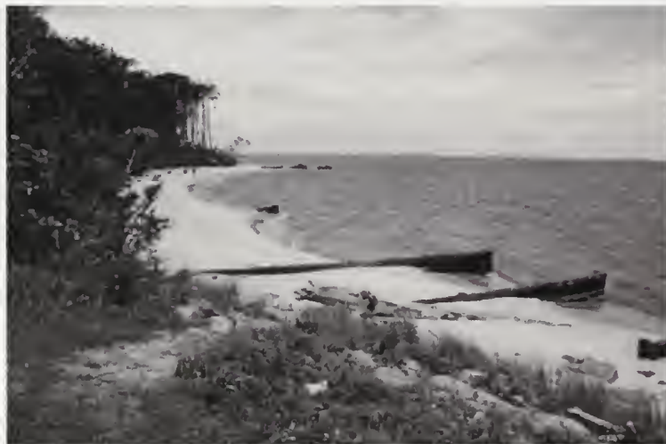
FIGURE 16. These wood groins have been constructed along the shoreline to control erosion. Source: JMA, Inc., 2009.
