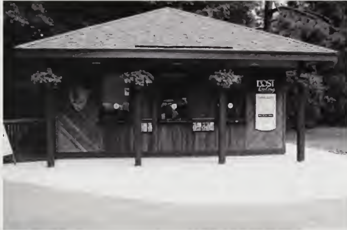
FIGURE 82. Building with signage. Source: JMA, Inc., 2009.
