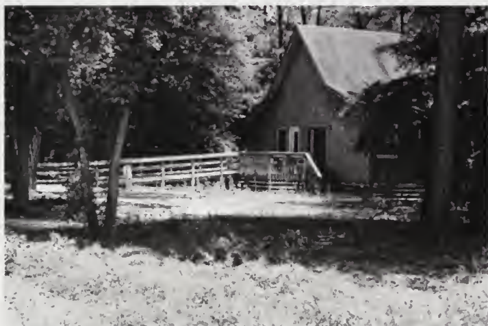
FIGURE 48. Wood frame building adjacent to the maintenance yard. Source: JMA, Inc., 2009.
