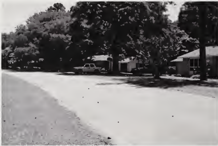
FIGURE 21. Cluster of staff housing along Pear Pad Road. Source: JMA, Inc., 2009.
